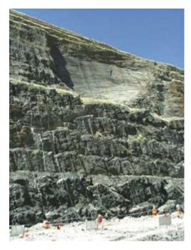
22. The highwall at your quarry has experienced a substantial failure of ground, which included the failure of two benches located at the top of a 5-bench face. You are undertaking a review of the current design parameters, possible causal factors and the development of a program of works to continue mining.
