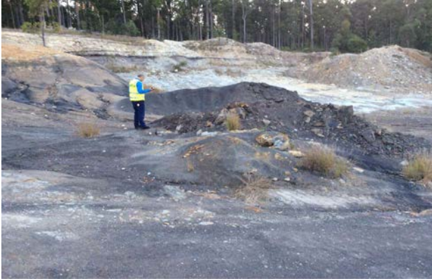
Figure 3 Before – disturbed areas in the pit floor, including waste material stockpiles, were the source of potential offsite pollution during storm events due to sediment laden run-off
