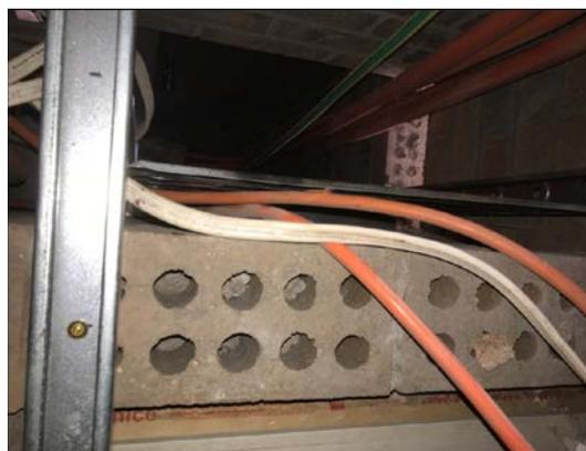
When working in confined areas like roof spaces where electricity is present, an engineering risk assessment must be completed and all energy sources need to be identified and appropriate isolation controls implemented.
