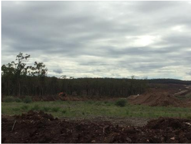
Figure 9 Northern clearing area - topsoil and gypsum stockpiles
