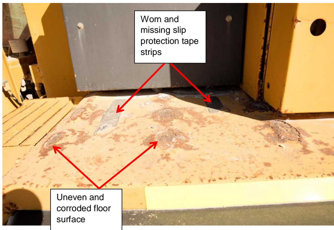
Figure 11: A closer view of the degraded condition of platform (position number 8) leading onto top of steps.
