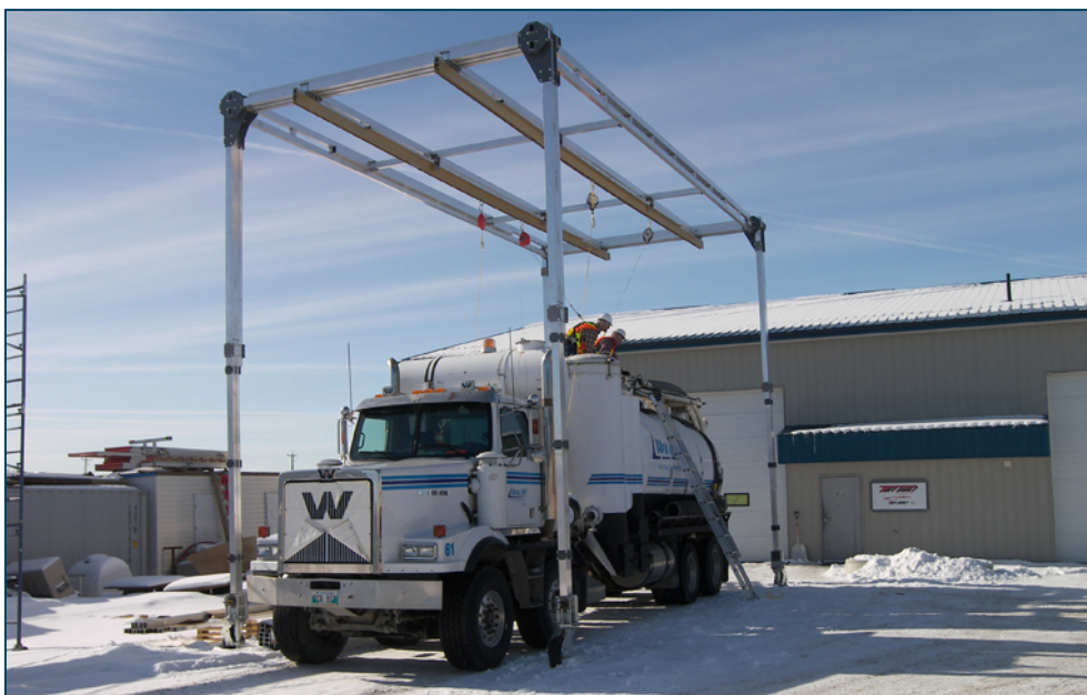
Figure 30: Example of a fixed fall arrest system. (Internet photo)
