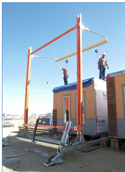
Figure 32: An example of a mobile fall arrest system. (Internet photo)
