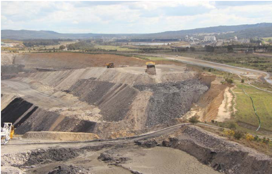
Figure 3: Northern highwall failure remedial works 18 September 2015.
