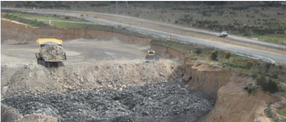
Figure 5: Northern highwall failure remedial works at 5 October 2015 showing failed area backfill completed.
