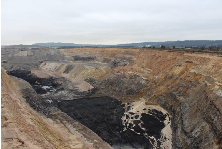
Figure 2: Northern highwall failure remedial works 15 June 2015.
