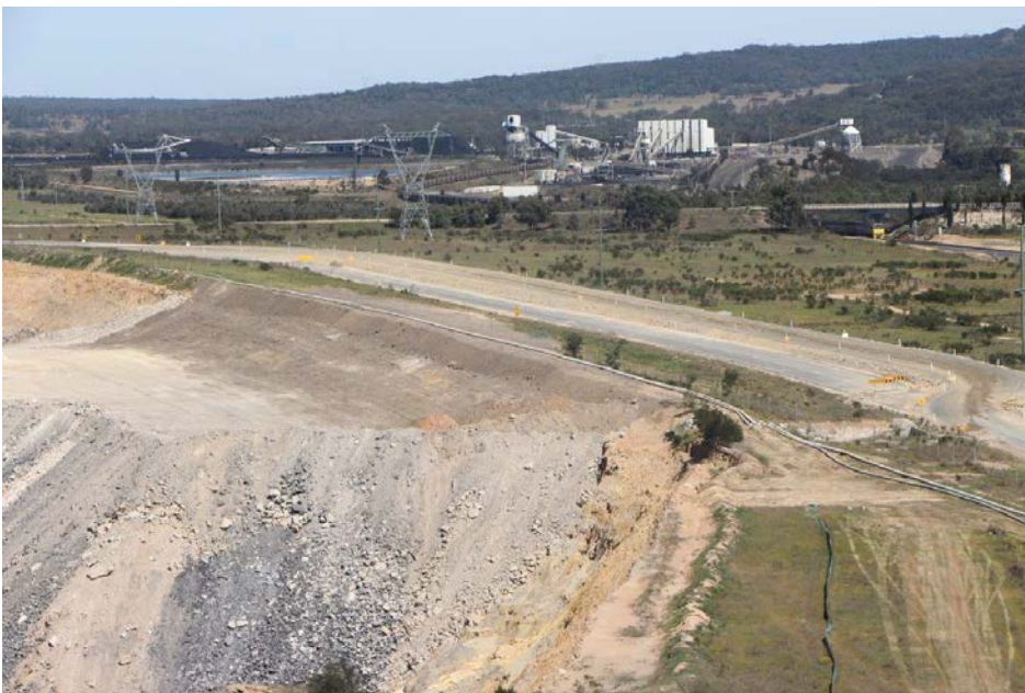
Figure 5: Northern highwall failure remedial works at 5 October 2015 showing failed area backfill completed.
