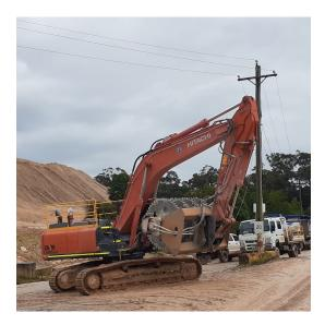
When developing roads or other vehicle operating areas, the potential for interaction between mobile plant and fixed structures, such as overhead power lines, must be assessed. Controls must be put in place considering the hierarchy of controls in accordance with Work Health and Safety Regulation 2017 clause 36 Hierarchy of control measures
