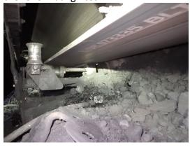
Workers conducting inspections on conveyors must diligently inspect for fire risks such as accumulation of coal, failing or collapsed idlers and contact between conveyor belts and fixed structures.
