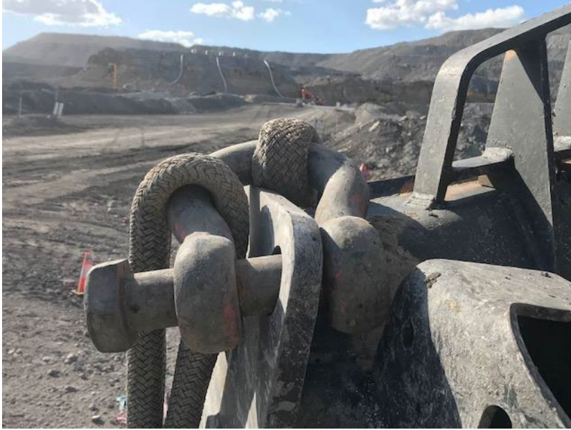
Figure 3: D-shackle connecting sling 2 to D10 dozer blade tow/lifting point
