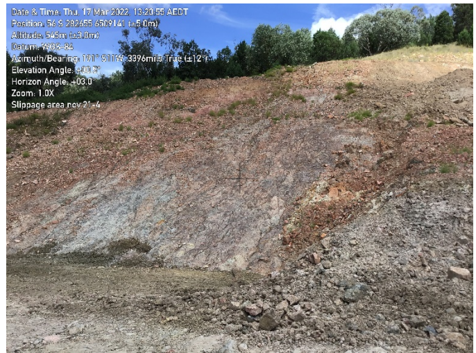
Figure 4 Chocked area to stabilise slippage
