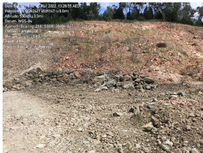
Figure 4 Chocked area to stabilise slippage
