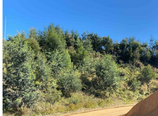
Figure 12 Rehabilitation of bund west of western stockpile area
