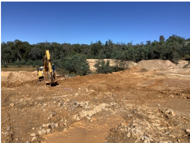
Figure 13 Backfilling and compacting of sediment basin 1 (SB1)
