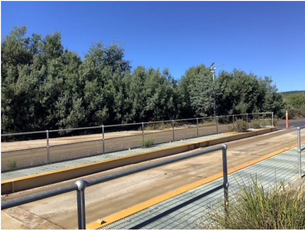
Figure 14 Natural revegetation of batters south of the weighbridge
