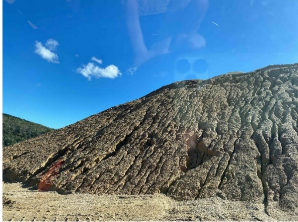
Figure 6 Erosion rilling evident on stockpile
