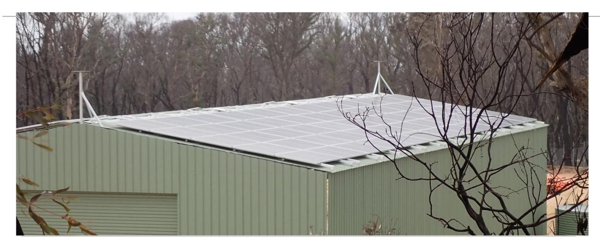
Off grid system – 120 cells (3 phase system with batteries and a generator back up) No access possible up the roof along the edges (but accessible by EWP).
