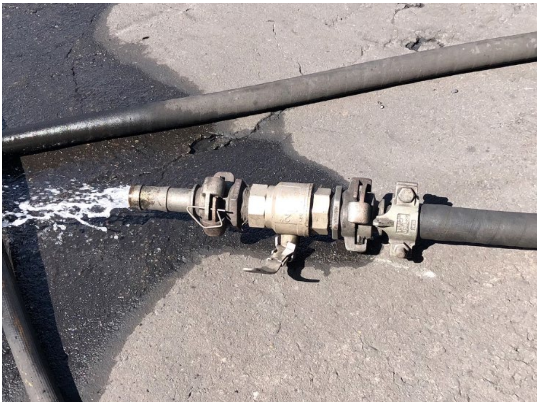
Figure 1: Ball valve with lever handle fitted to the free end of a hose at a mine
