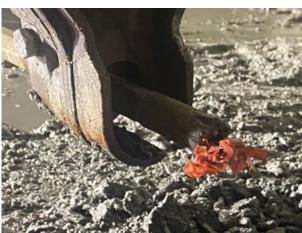
Mine operators should have a process where drill holes are checked, and any misfires cleared, before the next pattern is marked and drilled.
