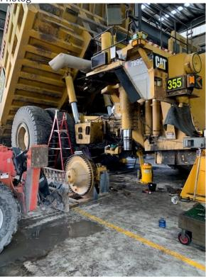
When removing components that may release instantaneously (such as those on a taper), controls must be in place to protect workers from the sudden release of energy. This may include using a boss and retaining bolts, timber packing, restraining slings or strops. If forklifts and telehandlers are used, the impact of pneumatic tyres and boom extension should be considered when assessing movement of the load.
