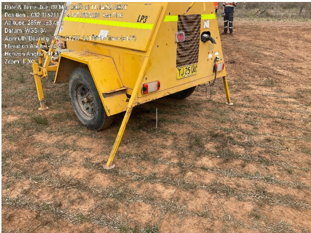
Figure 1 Lighting plant with no spill protection underneath
