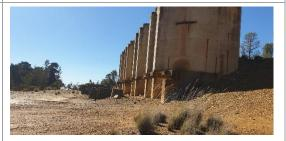
Derelict concentrate bins with sulfidic waste and water seepage
