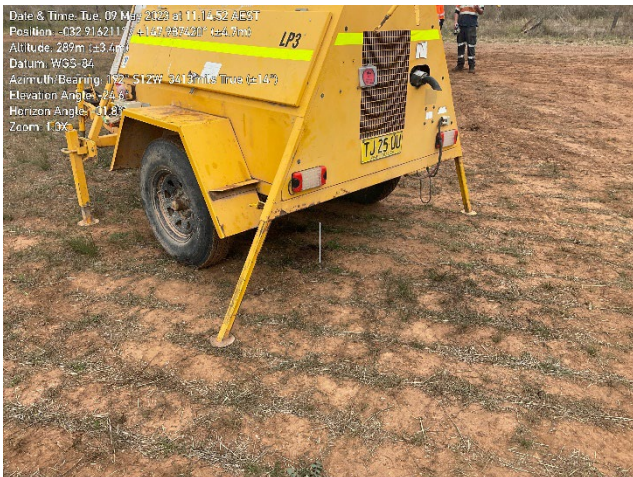
Figure 1 Lighting plant with no spill protection underneath
