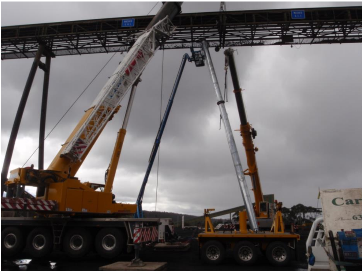
Figure 1: Leg assembly resting on elevated work platform
