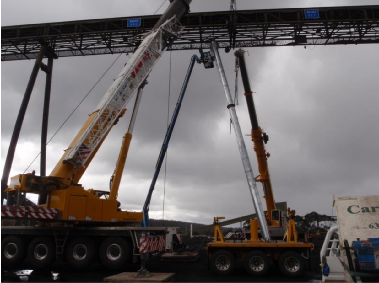
Figure 1: Leg assembly resting on elevated work platform
