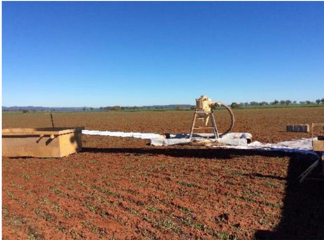
Figure 3 Return water discharged through geomatting into the paddock
