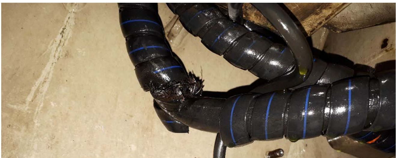
Figure 11 Bengalla fire incident
