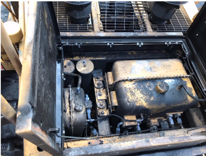
Figure 274 Rix’s Creek incident
