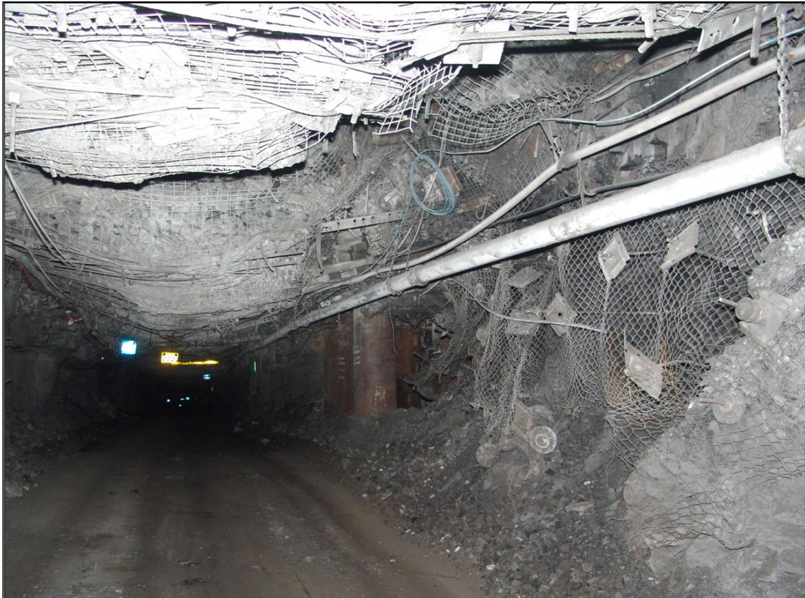
The above photograph shows a roadway that has undergone convergence, been re-supported and is now stable. There will obviously be voids in the roof and ribs, resulting from the convergence, that allow the movement of a significant quantity of air across a stopping or seal placed in the roadway. Strata injection or sealing of the strata is necessary in these circumstances to provide effective containment.
