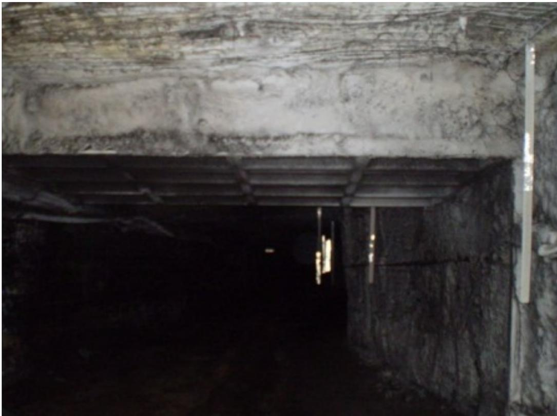
Attached to the door is a manual winch, operated from the surface of the mine but which can also be configured to be operated from a location within the mine such as an outbye cut-through etc. The door resides in the open position & if required, (emergency), the winch firstly lifts the door slightly & the roof latches let go & allow the self-locking door to be lowered to seal the area.
