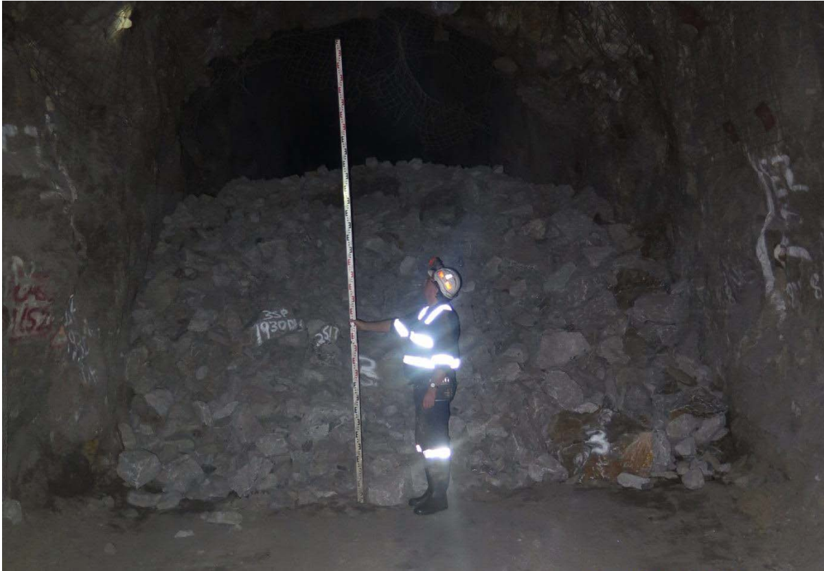
Figure 3 – Proposed method of controlling bund heights, courtesy of Perilya Ltd.
