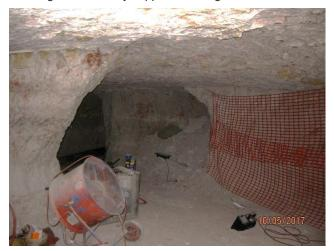
Primary support is the support required to hold up the mass of ground between the underground mine workings and the surface. Only pillars are capable of providing primary support.
