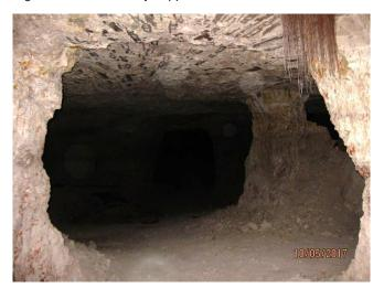
Figure 5: No secondary support installed.
