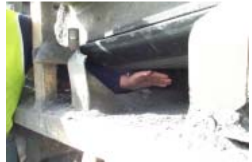
Photo shows unguarded conveyor
