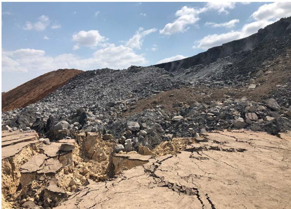
Figure 2 Recent highwall failure January 2020
