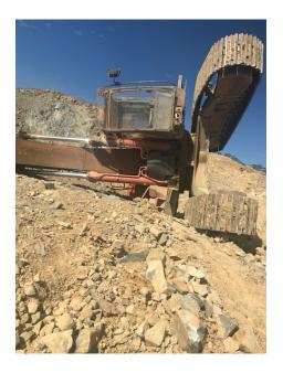
Dangerous incident SinNot-2018/00554 A highwall failed and material spilled over the bund protection and onto the working bench below. This blocked access to part of the pit. While no workers were present in the area where the failure occurred at the time and no equipment was damaged, three workers were temporarily unable to egress the pit due to the access ramp being damaged when the highwall failed.
