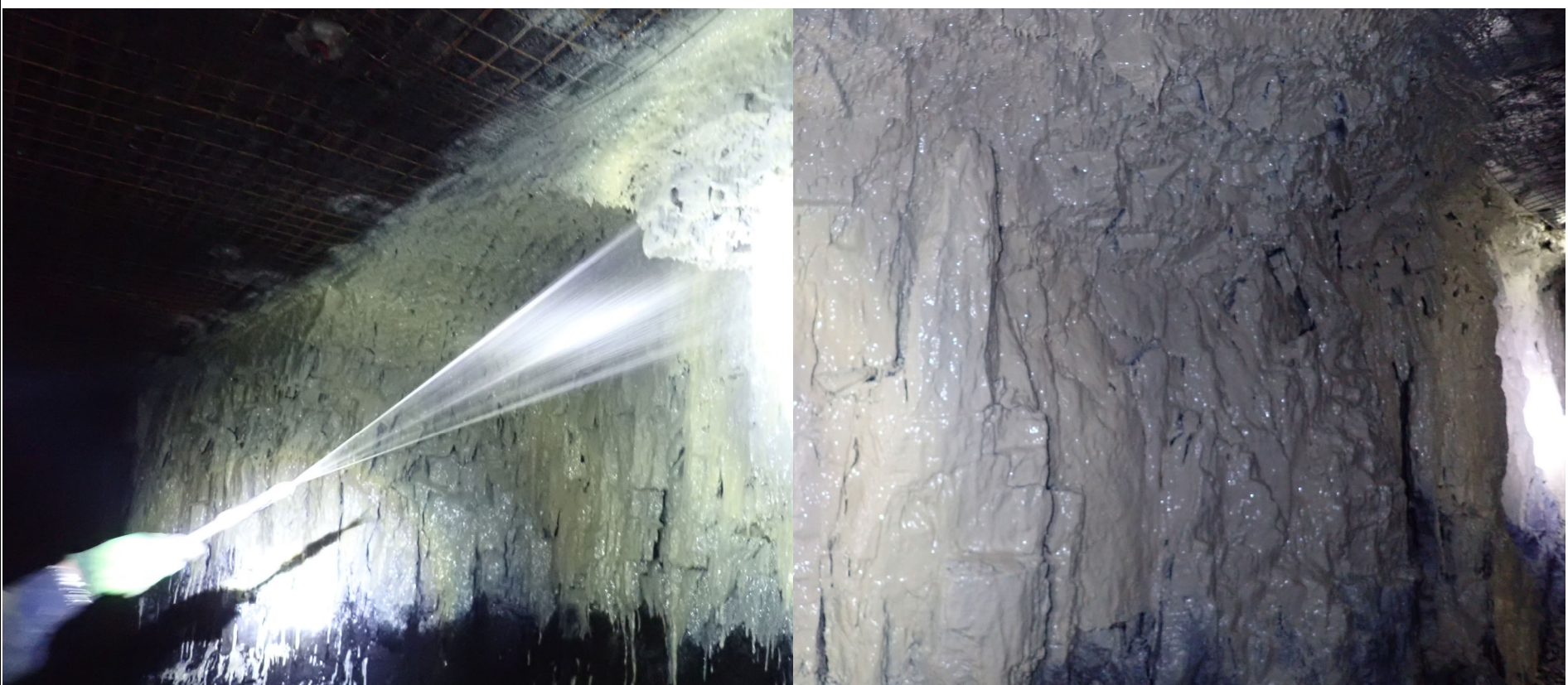
Figure 16c: Subsequent Coats being Applied
