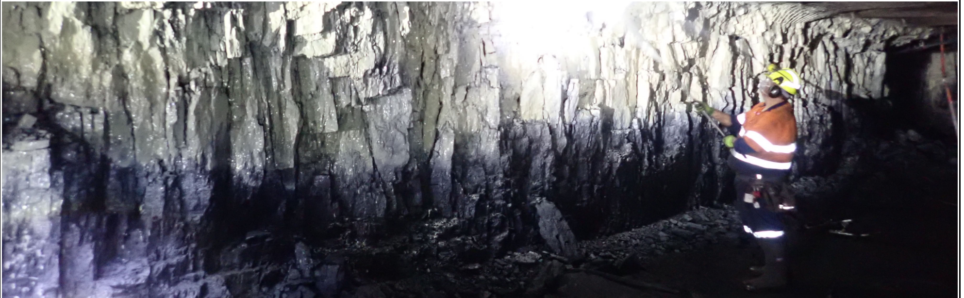
Figure 16b: First Coat being Applied
