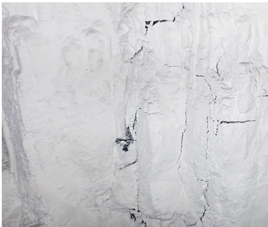
Figure 18c: Localised Dilation on Pre-Existing Discontinuities (Cleat and Bedding) - Inbye Rib of 0.5C/T, A to B Heading
