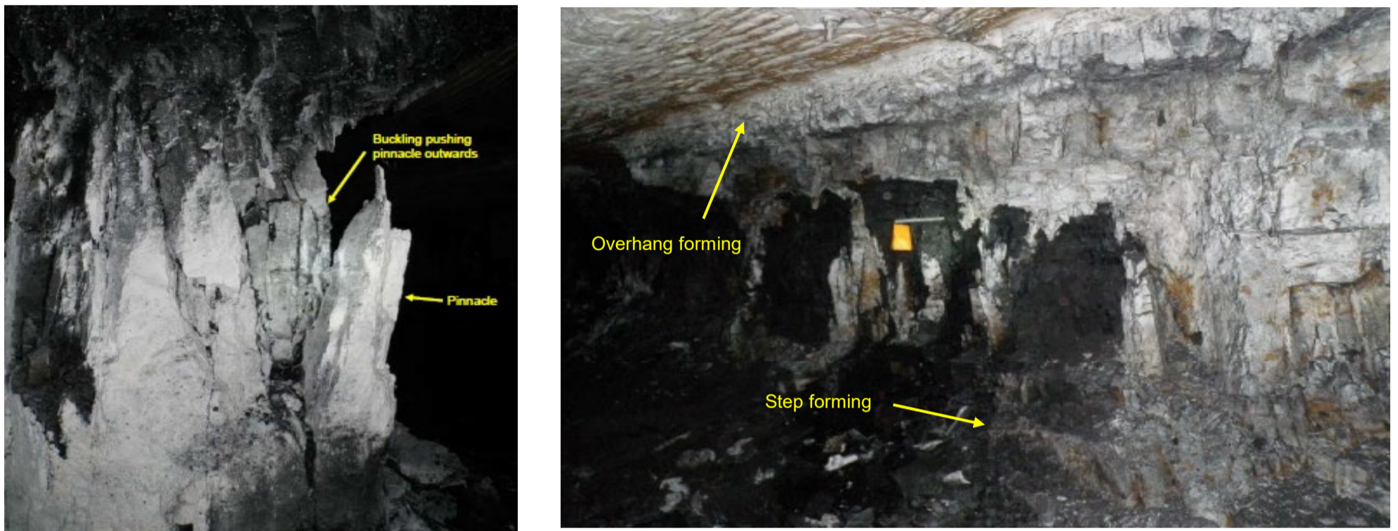
Figure 9b: Behaviour of Unbolted Ribs in the Older 400 and Outbye 900 Areas of Clarence
