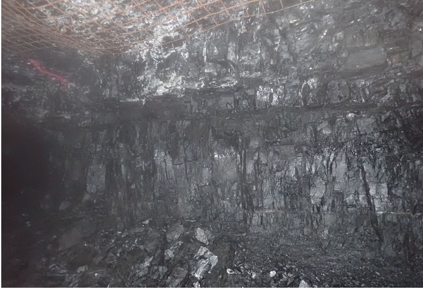
Figure 16a: Washed Down Rib prior to Sealing
