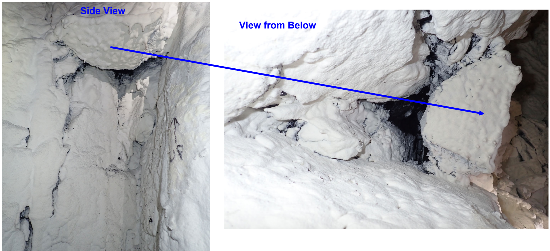
Figure 18c: Localised Dilation on Pre-Existing Discontinuities (Cleat and Bedding) - Inbye Rib of 0.5C/T, A to B Heading
