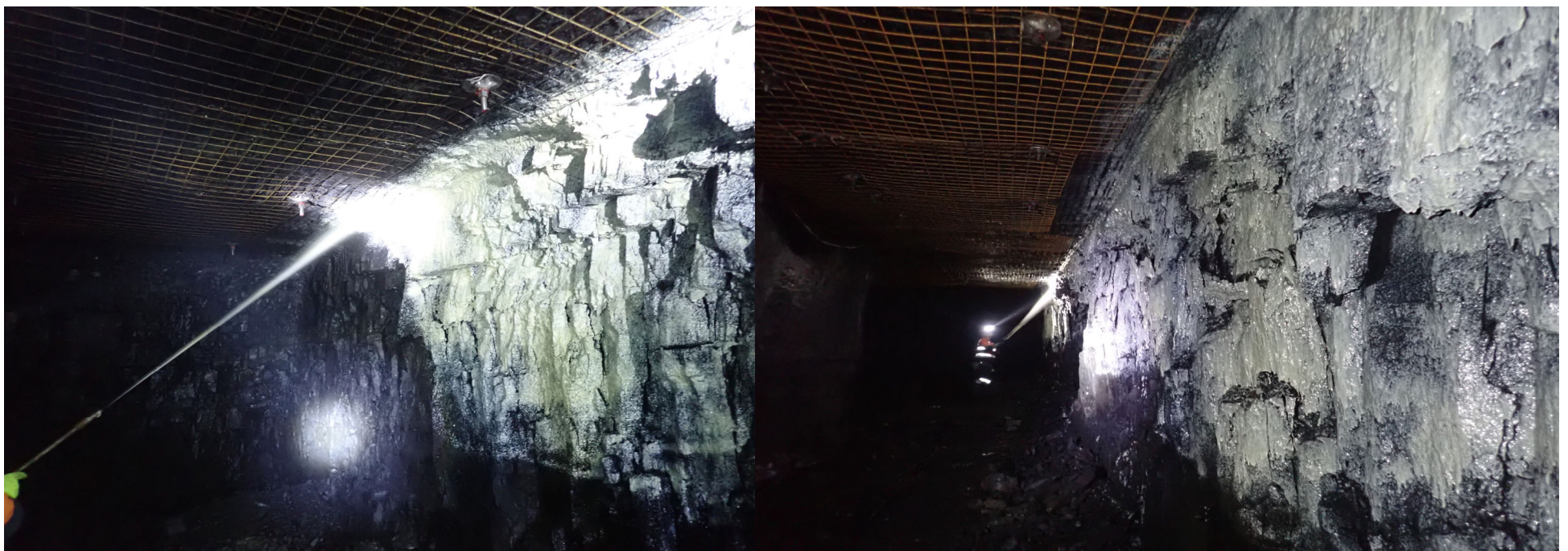
Figure 23b: Spraying of the First Coat
