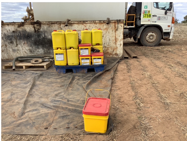
Figure 2. Drilling chemicals, fuels and oils on bund over tarp
