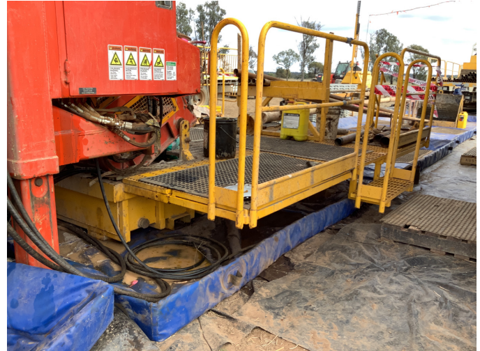
Figure 5. Drilling platform and trough
