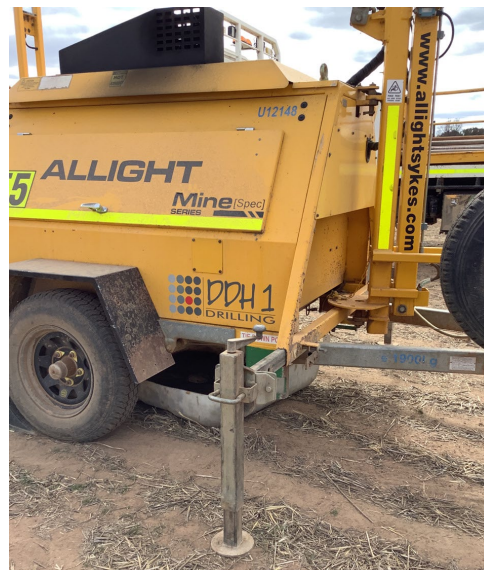
Figure 4. Spill containment under lighting tower
