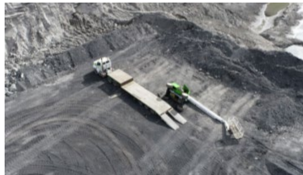
Above: The elevated work platform and loader.
