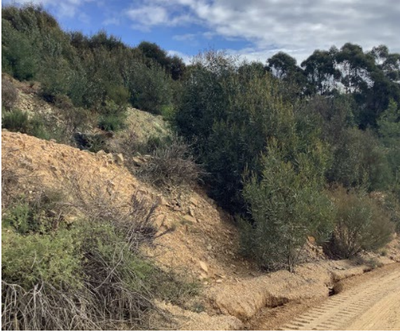
Figure 11 Bare areas along the benches
