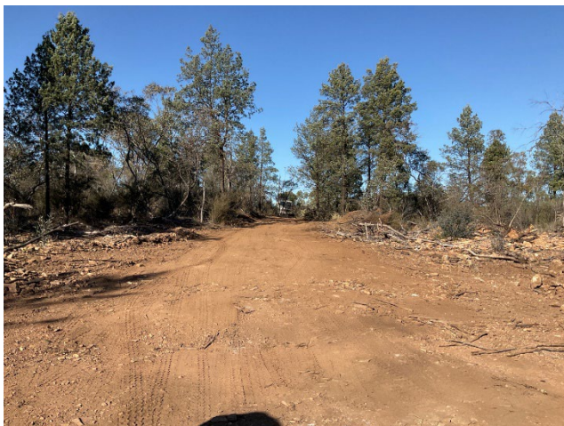
Figure 3 Short section of track pushed in to access drill pad TBRC66
