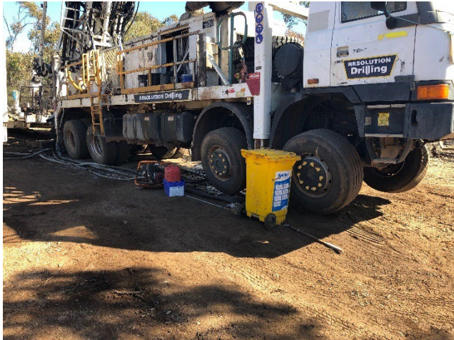
Figure 2 Spill kit, rig nappy, and secondary containment for pump fuel container at the diamond drilling site
