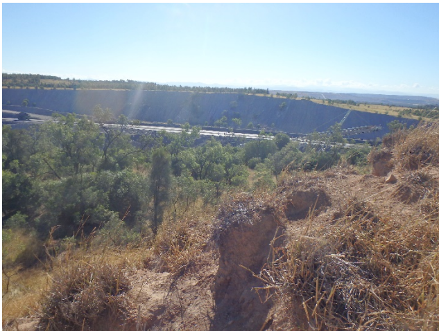
Figure 3 Stockpile 7 showing steep eroding batters
