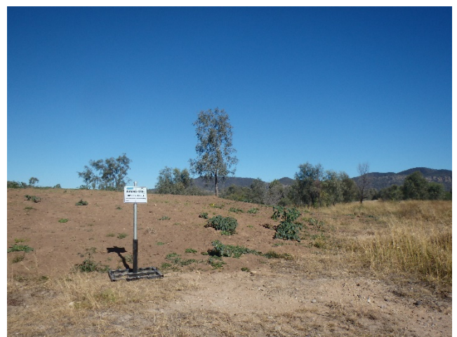
Figure 6 Lack of cover crop establishment on stockpile 5
