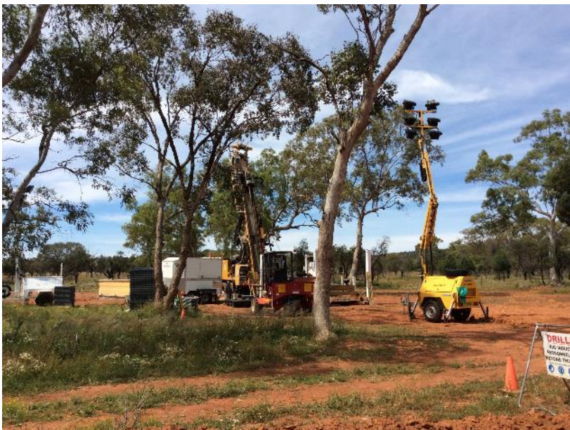
Figure 6 Diamond drilling at 20BMDD011
