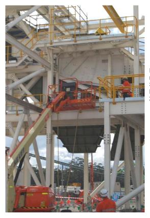
Figure 41: View of the platform outside of the second floor main frame and being lowered vertically past the first floor. Spotters relocated to the first floor area and the ground level. Photo taken during lowering of the platform on 23 May 2014. Figure 42: View of the platform outside of the main frame and being lowered past the first floor. Spotters relocated to the first floor area and the ground level. Photo taken during lowering of the platform on 23 May 2014.
