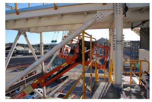
Figure 36: Platform and articulating jib position in relation to the stairway handrail.
