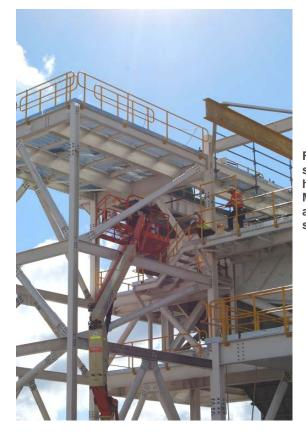
Figure 39. View of the platform moving parallel with the steelwork and lowered adjacent to the walkway steps handrail. Photo taken during lowering of the platform on 23 May 2014. The spotter is on the second floor walkway. The articulating jib and main boom have moved closer to the steelwork of the structure.
