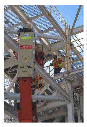
Figure 38. View of the base boom, upright and main boom position in relation to the second floor and third floor horizontal steels, the angled cross brace connecting floor the two floors and the handrail of the second floor walkway. The spotter is standing on the second floor walkway observing the platform movement controlled from the ground control box. Photo taken during lowering of the platform on 23 May 2014.
