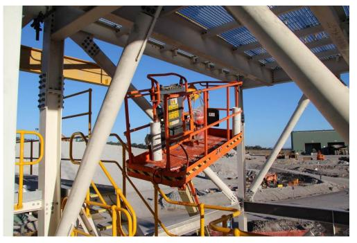
Mr Galton, 51, was relocating the platform to ground level after tightening bolts on the structure. During the movement of the platform over walkway handrails, a crush point was created between the platform frame above the control console rising towards the steel beam. Mr Galton was alone in the platform.
