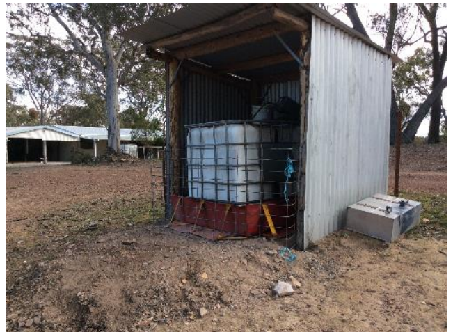
Figure 4 Bunded waste oil storage
