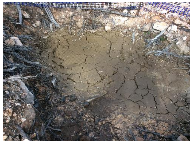
Figure 4 Sediment left to dry out before backfilling at BD20-001
