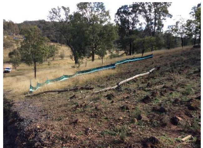
Figure 8 Salvaged vegetation and sediment fencing at rehabilitated site BRC17-019
