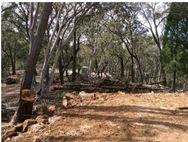
Figure 5 Blue flagging tape to mark drill pad site
