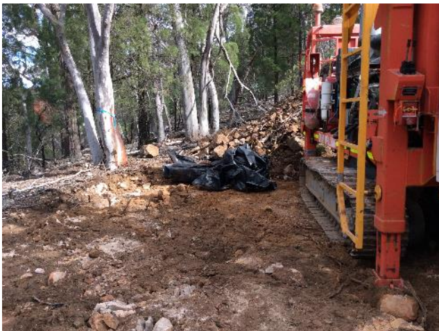
Figure 3 Rig nappy ready to be placed under drill rig
