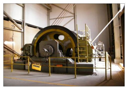
Figure 24 Tower mounted friction winder showing two brake paths
