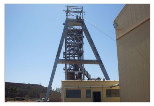
Figure 14 Headsheave installation - drift winder
