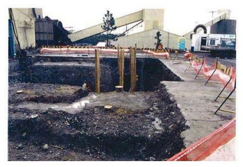
Figure 10 Winder foundations showing pit and footings
