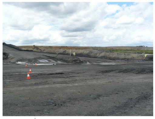
The intersection and the 8<sup>th</sup> ramp were built between 25 July 2012 and 19 August 2012. The 8<sup>th</sup> ramp was modified between 24 August 2013 and 22 September 2013 when a coal ramp to the stockpile was established. Before July 2012, there was an intersection and haul road further
