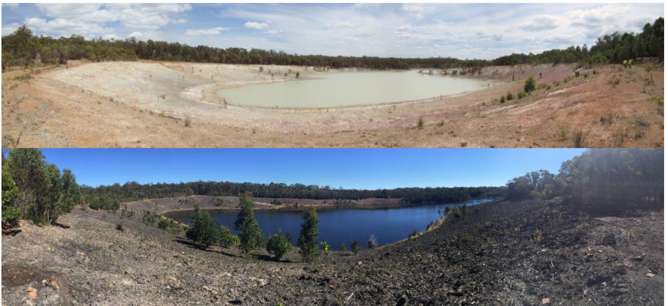
Figure 11 Rehabilitation progression – final void from 2015 to 2019
