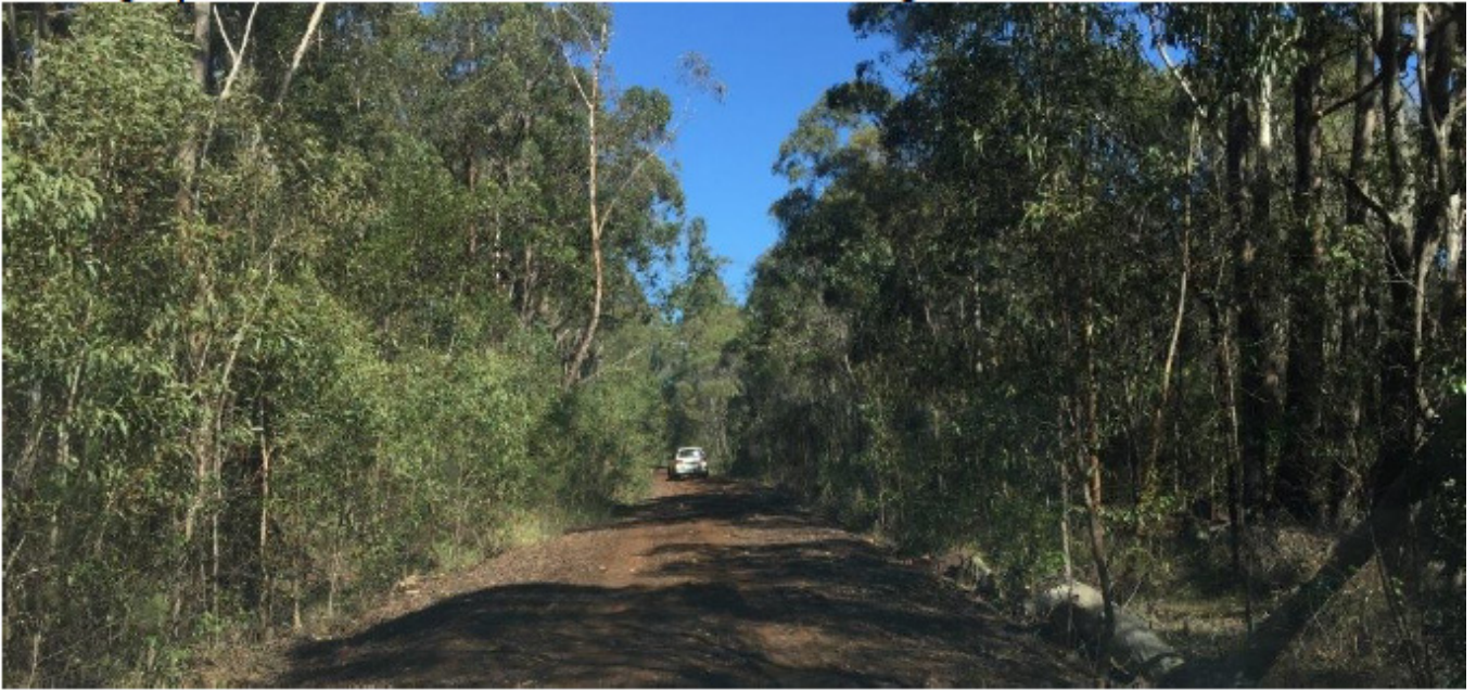
Figure 5 Access road remaining on the site
