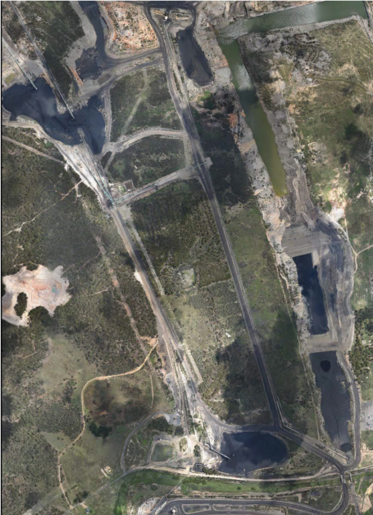
Figure 5 Rehabilitation status in 2019
